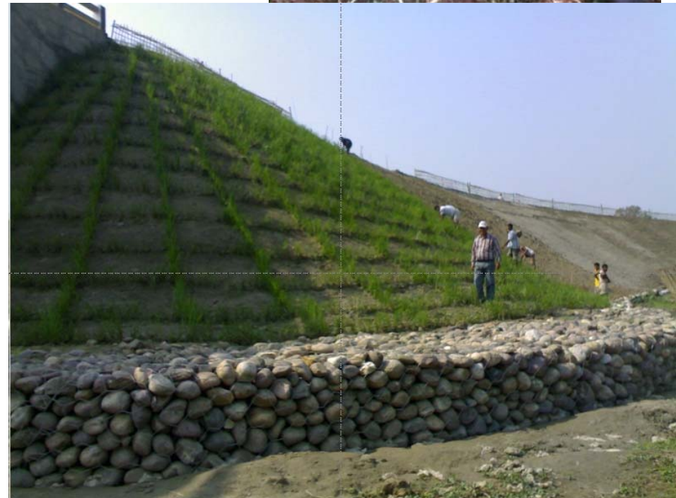
The forward slope toe protected with caged boulder
